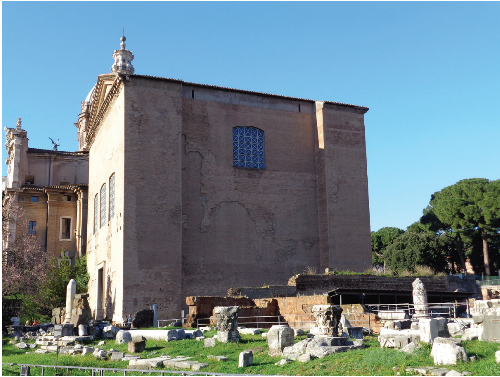
Fig. 7. Roman Senate House (Sant'Adriano), Rome, exterior (photo by author); reconstruction of interior (photo from ULCA Digital Forum)
